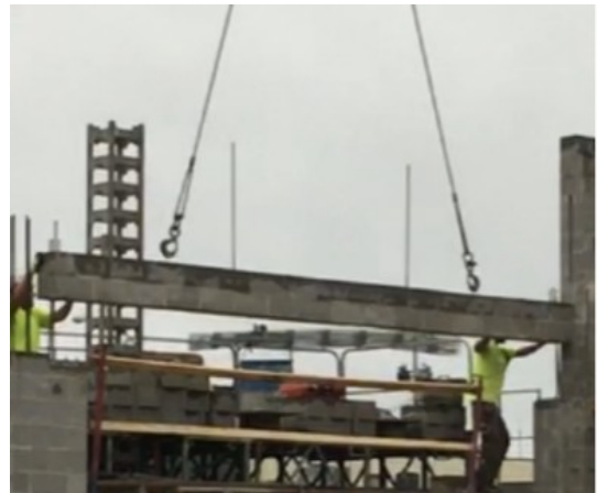
Figure 1: Prefabricated Masonry Lintel
